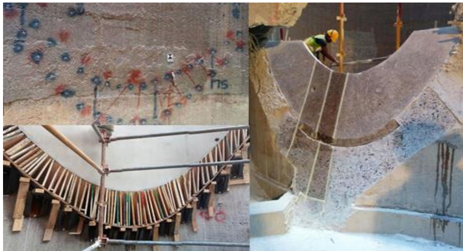
Figure 14. Zeitz MOCAA: Marking for cutting existing silo surfaces.
