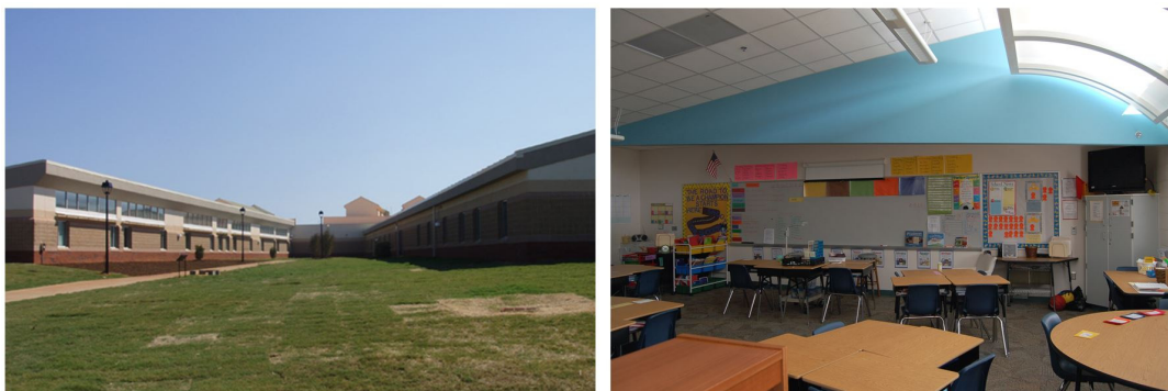
Figure 1. Reedy Fork Elementary School.
